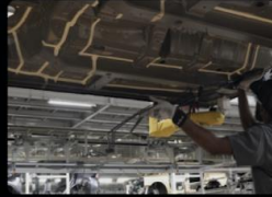
Fuel and brake line installation
