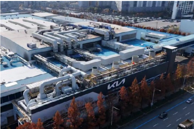
Installation of eco-friendly concentrated RTOs
